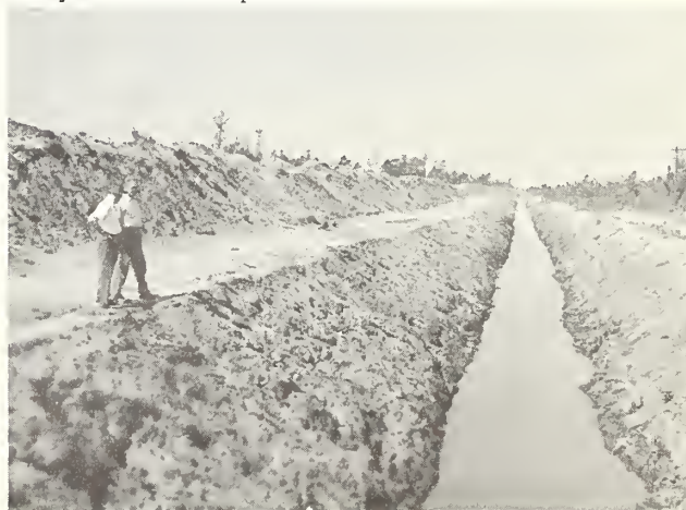
MAIN DRAINAGE CANAL - Good alignment and spoil management.
